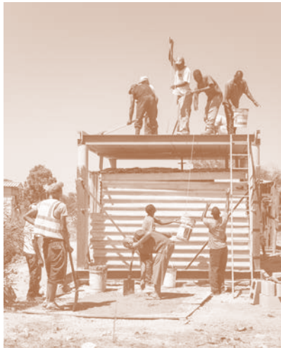
Construction process—various actors participating in the construction of the prototype
