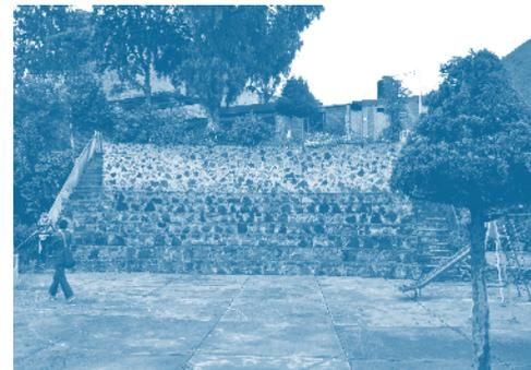
The kindergarten in Miravalle is a good example of the community's ability to create pleasant and multi-functional spaces, taking advantage of topography and local resources. Located on a steep slope, teachers and parents used volcanic stones to build a retaining wall, with steps that double as seats for the open-air amphitheater.
